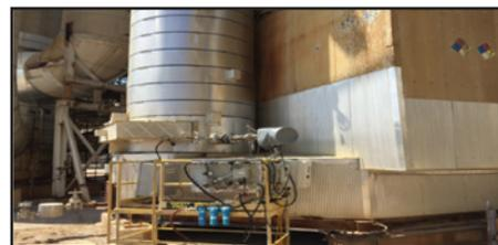
Fig. 3: Breen-SA Probe Rev 2 installation.
