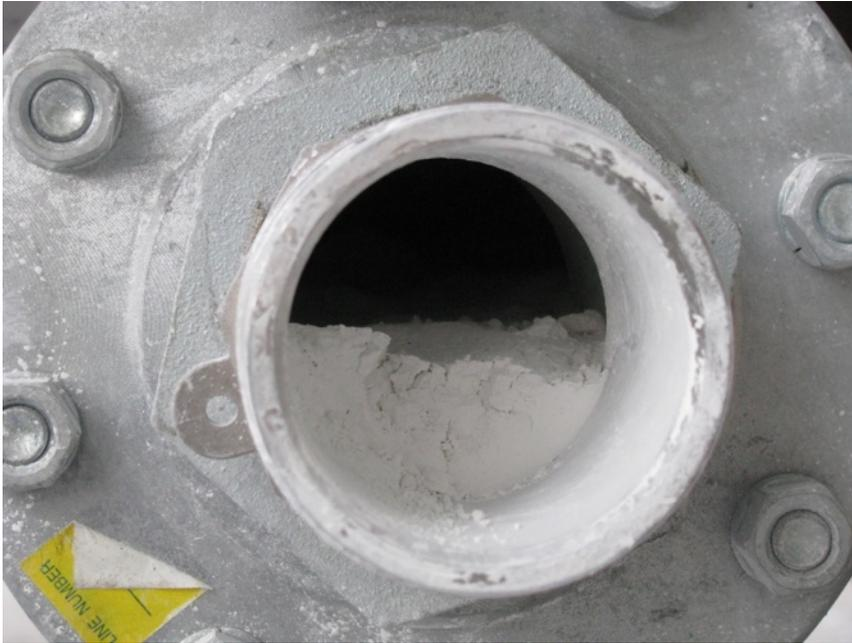
**Figure 8 - Outlet of the Transition Chute below the Feeder after 38 days of operation**
