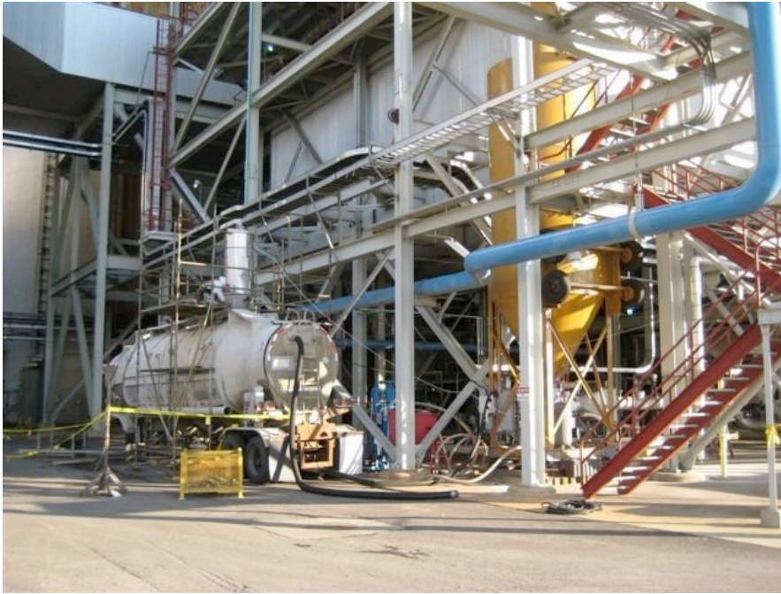
Figure 6 - The Equipment Installation at Site
